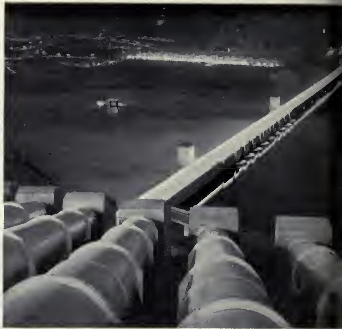
WORLD'S LARGEST PUMPS (above) lift water 280 feet out of the Columbo River, into the Feeder Conol. Farther south the water is held behind Long Lake Dom (ot left). Brook Lake in the foreground. Photo above by H. W. Fuller, ot left by F. B. Pomeroy, both Region 1 photographers.
